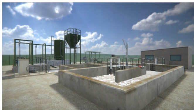
Figure 1: A snapshot of the immersive Digital Twin - biological reactor at the San Esteban de Litera Wastewater Treatment Plant.
